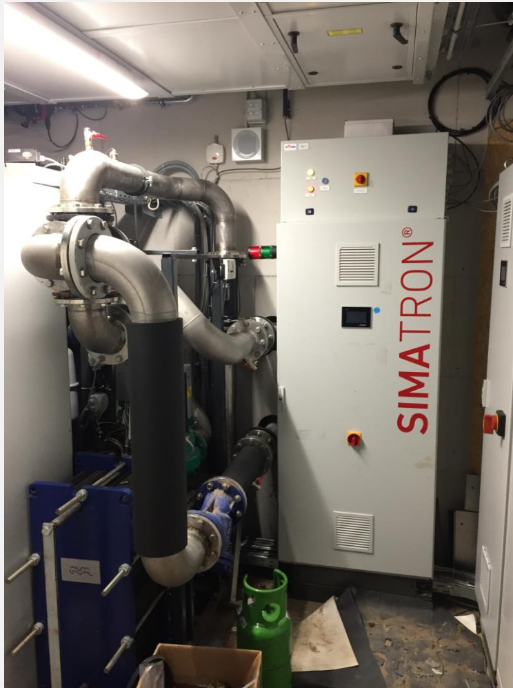
Figure 17: Heat pump and heat exchanger Sportscomplex (October 2018).
