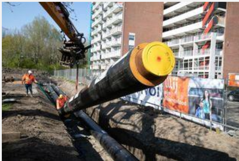
Figure 14: Construction of heating grid next to Nijestee flat 1.
