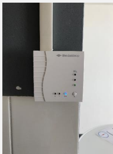
Figure 3: CO 2 ventilation controlled ventilation
